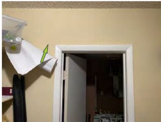
Photograph 135 Building 21; Unit 2123; Walk-In Closet
