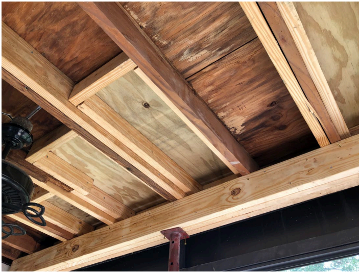
Temporary repairs and shoring to deteriorated framing at Building 22
