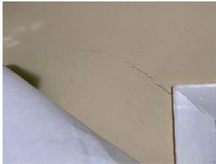
Photograph 136 Building 21; Unit 2123; Walk-In Closet
